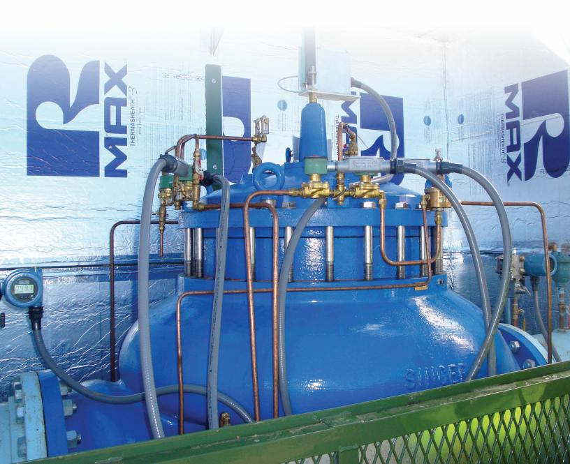
IN 2010, SINGER VALVE INSTALLED A FILL CONTROL VALVE ON A NEW 4 MILLION GALLON (15,141,647 LITER) STORAGE TANK. ANOTHER STORAGE TANK WAS IN CLOSE PROXIMITY AND CONNECTED ON THE SAME DISTRIBUTION PIPELINE, AND IT WAS CRUCIAL THE PIPELINE MAINTAIN NORMAL PRESSURE DURING FILLING CYCLES AS PRESSURE CAN DROP SUBSTANTIALLY IF BOTH TANKS ATTEMPT TO FILL AT THE SAME TIME.
